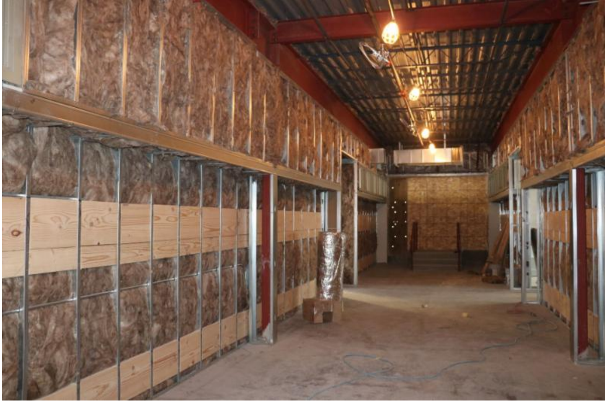
Inside the St. Mary's Grade School addition, progress is moving along with insulation, sheetrock, wiring, paint and more!
