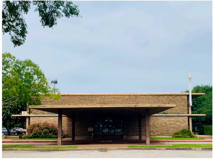
EAST SIDE BUILDING ENTRANCE
