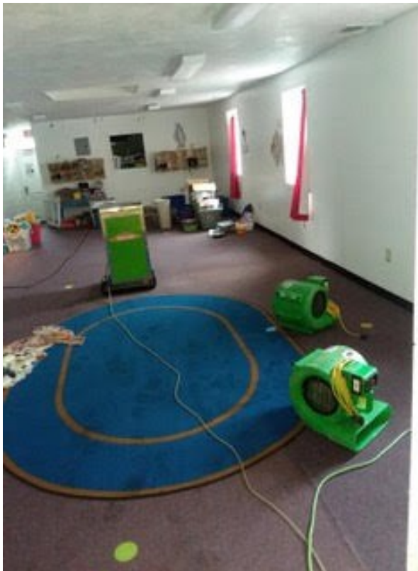
HFS Pre-school room at Griffin Hall remediation work
