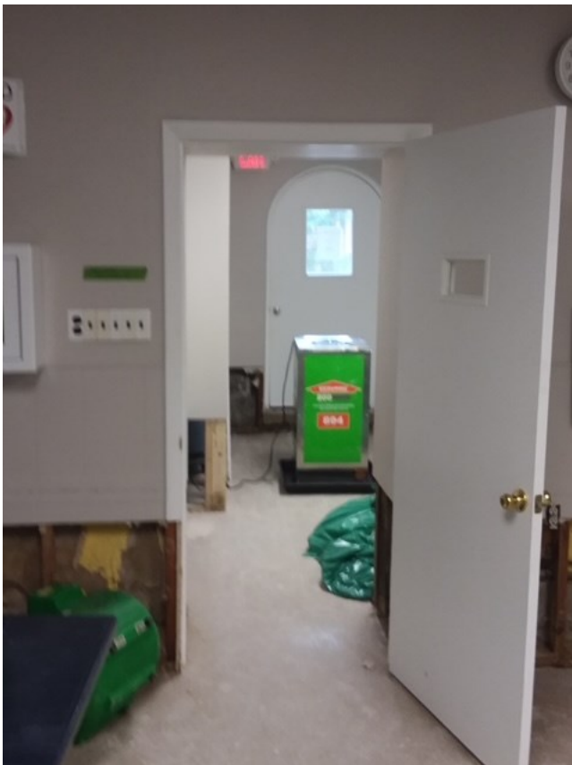
Church Hall remediation work, wet drywall was removed
