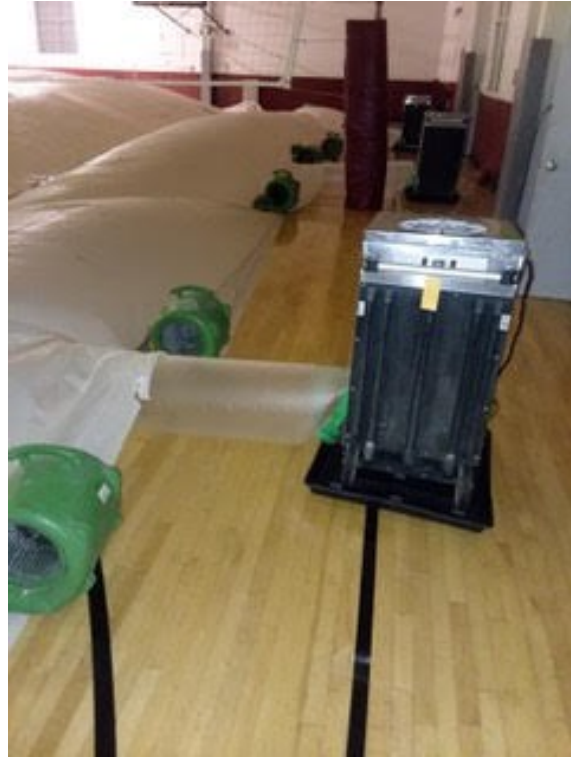
Griffin Hall remediation work, fans and dehumidifiers
