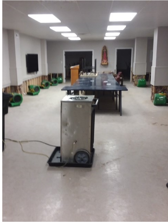
Church Hall remediation work, fans and dehumidifiers
