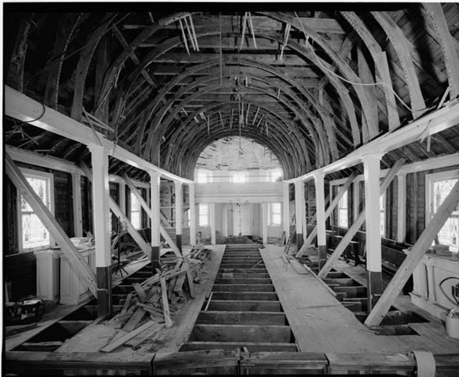
Restoration of St. Francis Xavier Church May 1983
