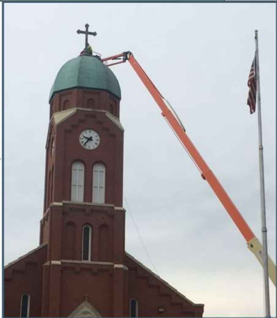
Lightning Rod Installation
