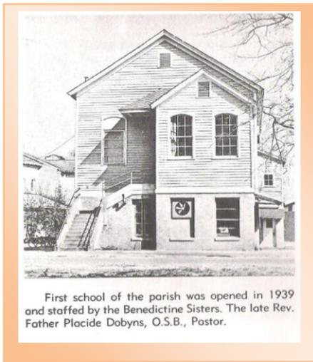
The old wooden frame church was moved to Avenue C and elevated to become a second floor with a ground floor of brick supporting it from below. This composite building served as four-room school from 1939 to 1956 when, under Father Bordenave, the main building of the present school was built. The old school was then converted into a parish hall, dubbed Dobyms Hall, on the second floor and a school cafeteria on the ground floor.
