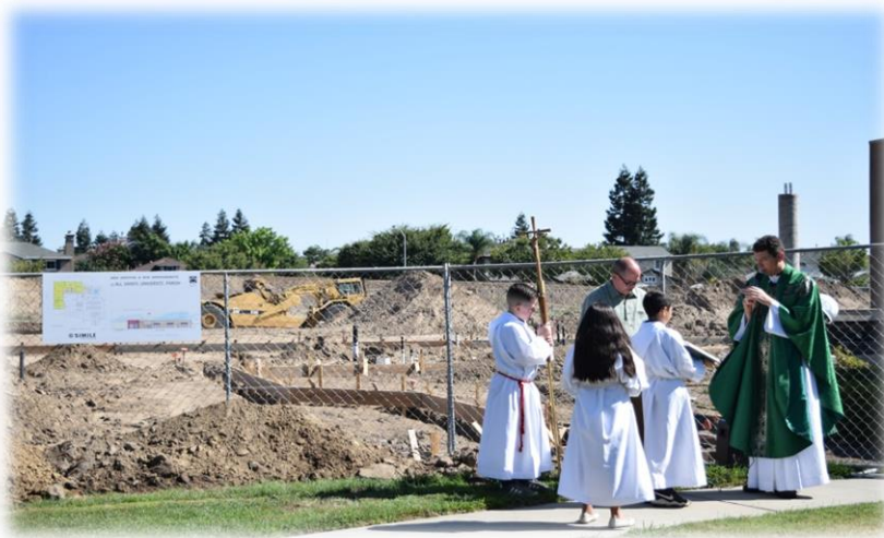
photo taken 7/28/2019 during the official groundbreaking ceremony for a new construction project that will allow for more room to meet and worship.
