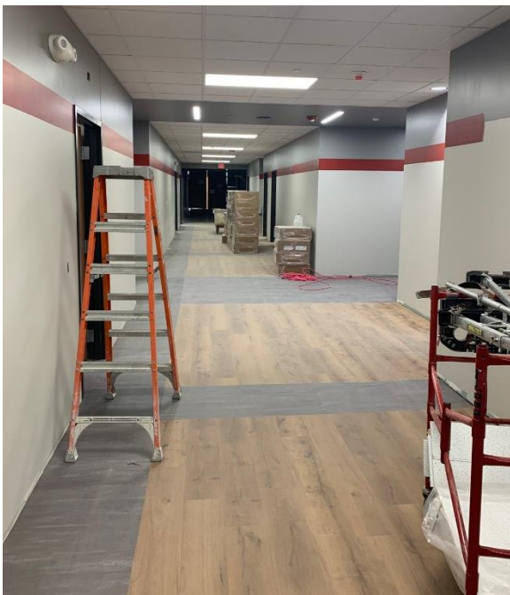
Main corridor on first floor
