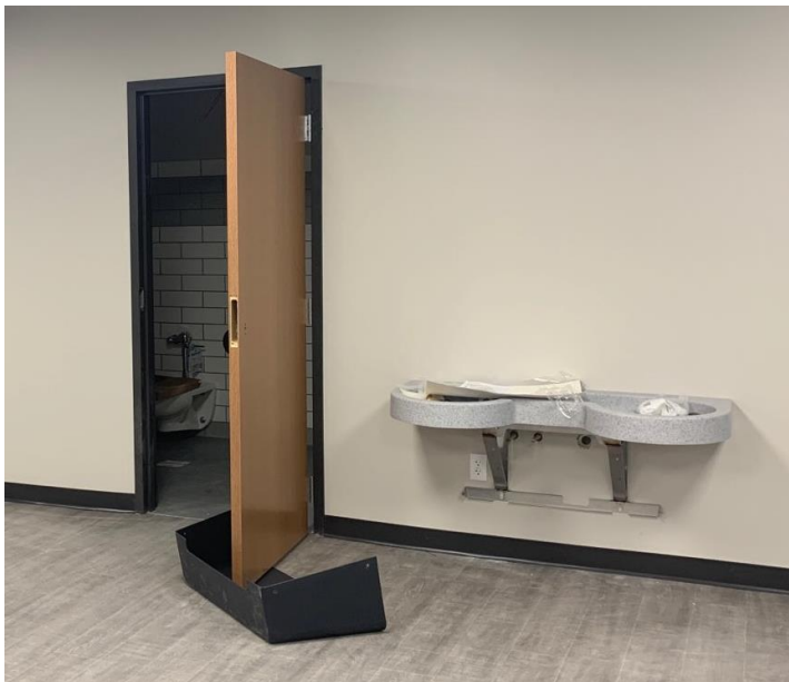
Lower level wash stations were installed
