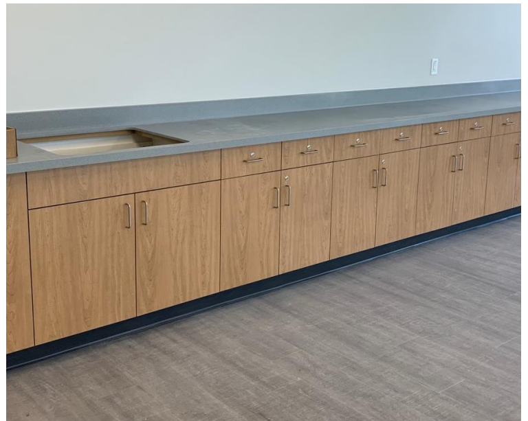
Art room casework and sinks are being installed
