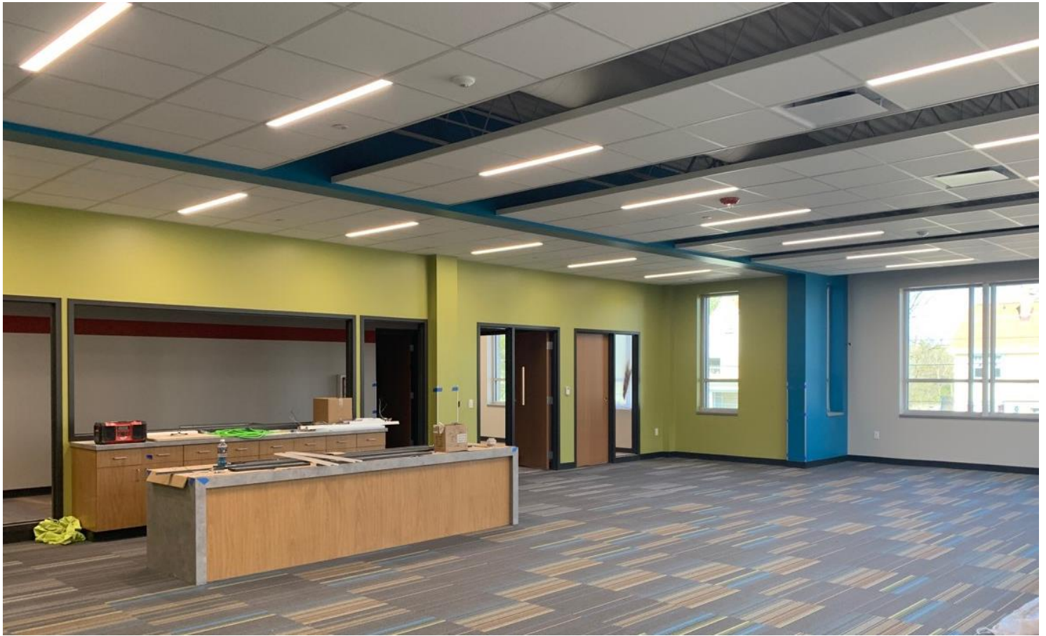
LMC light fixtures were installed this week
