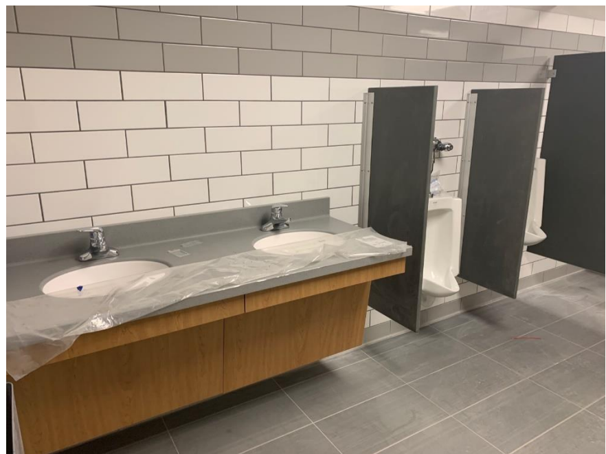
Sinks, toilets and urinal fixtures are being install on all floors.
