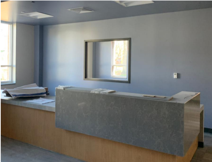
Admin area getting the final touches
