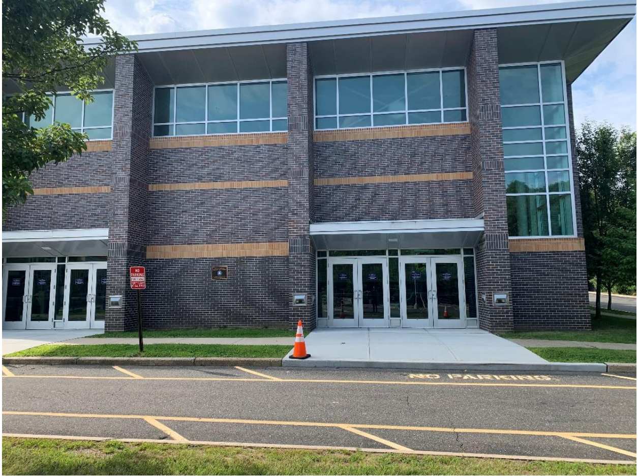
Handicapped Entrance to Weekday Mass (Gym Ground Floor)
