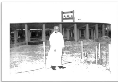
Msgr. Johnson and early church building
