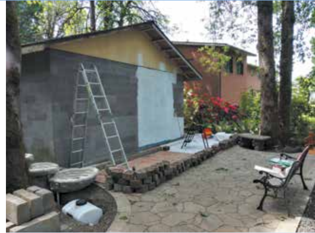
Photo taken during wall prep
