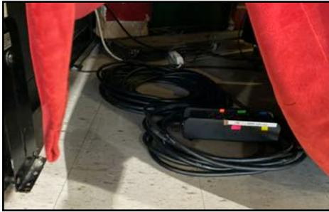
At the edge of the stage closest to the piano, you will find the end of the snake, with a bunch of microphone (xlr) inputs and outputs. There should be plenty of length in the small "puddle" of cable to bring the end of the snake to the piano, as pictured.
