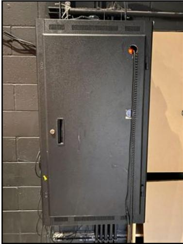
The gym sound system will also need to be on – it likely already will be on. That rack is in the opposite corner of the stage, mounted on the wall. The power switch is in a small hole on the upper right of the door (with some audio cables hanging out). If it's glowing orange, it's already on.
